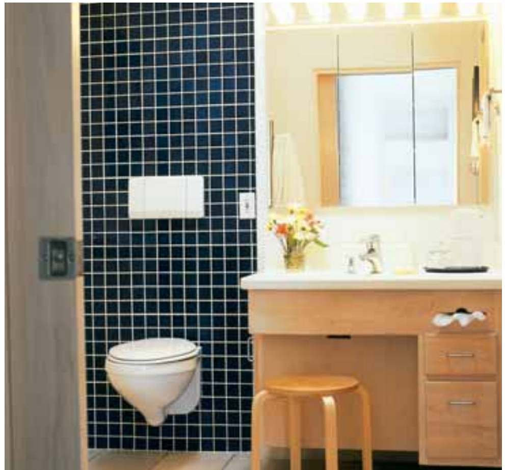
Suspended toilets in the bathrooms of the Pirkl house allow easy access and cleaning. Pull handles on cabinets and drawers permit easy retrieval of stored items.
