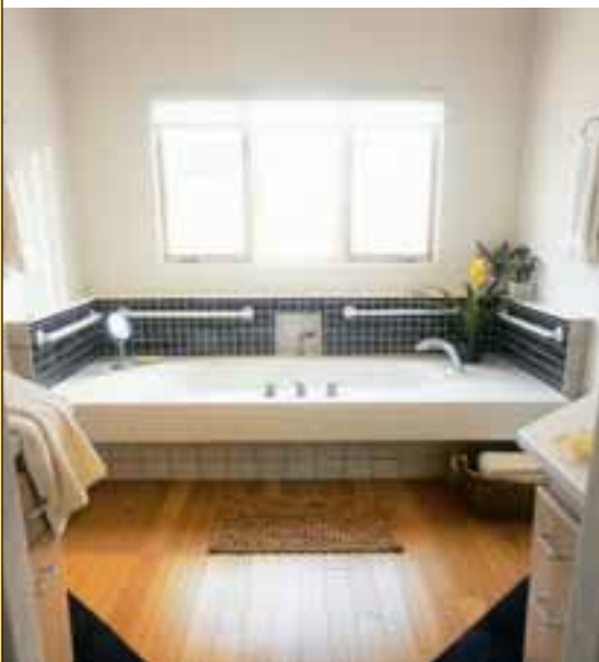
To eliminate slips, this soaking tub is surrounded by a wide tiled bench.
