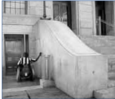
A new elevator entrance was provided next to the stairs to provide universal access to the services inside.
