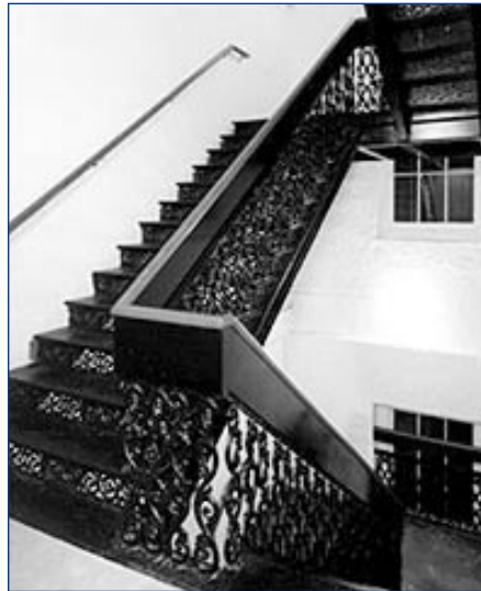
Example of a well-designed modification of a historic railing to comply with accessibility requirements.
