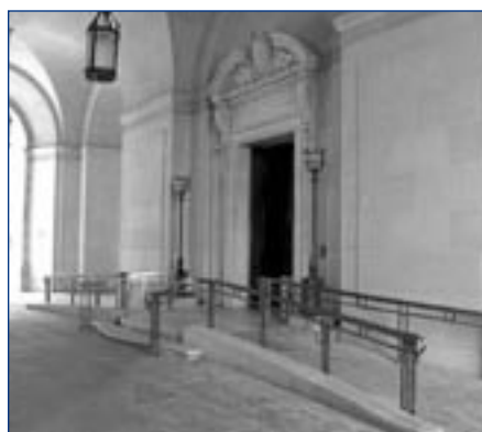
The ramps at this historic federal building were designed to provide equal access while preserving the building's original fabric.
